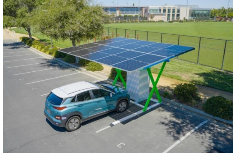
Figure 1: A solar-powered EV charging station canopy with integrated photovoltaic panels
